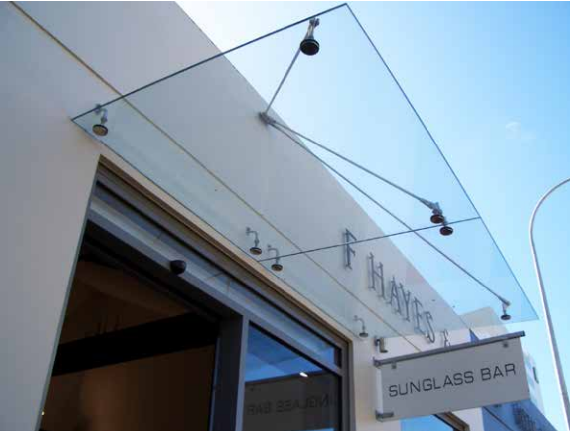
Specific Engineering design is required when tied back to a single fixing point.
